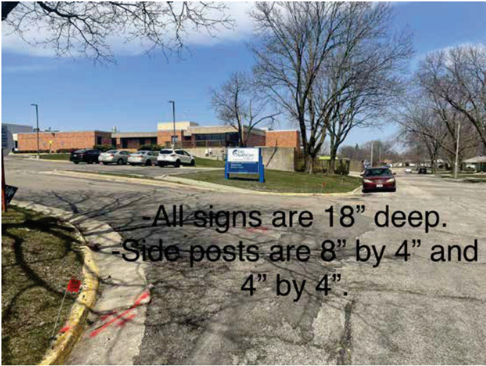
Existing Sign shown above replace with new Sign Type A - Medium Directional Monument: #S1
