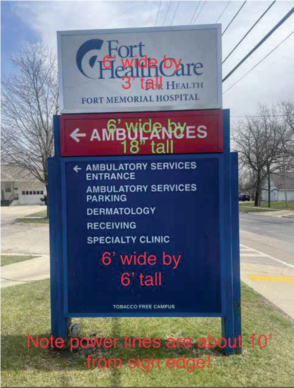
Existing Sign shown above replace with new Sign Type B - Large Directional Monument: #S2
